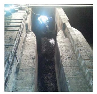
Figure 2: A large flume influenced by poor maintenance procedures allowing grit build up.
