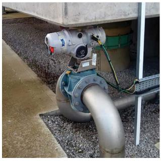
Figure 3 – Poor installation can breed poor maintenance. This control valve, installed underneath a raised tank, is not accessible for maintenance purposes.
