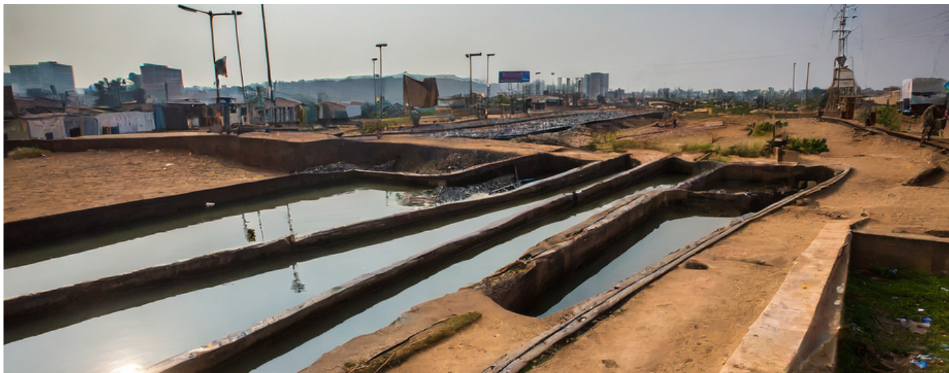
Sewer networks in a Sub-Saharan African city. Image generated on Adobe Firefly
